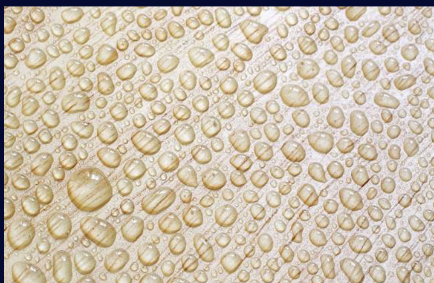
Figure 1: Sealant application of water-based polyurethanes
